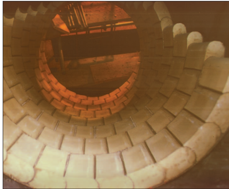
The above photo demonstrates book tile brick construction inside a drying tower.
