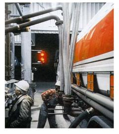
The main criteria of the loading arm are safe working, easy operation and maintenance. During filling there is adequate space between the loading arms and the tank truck. Giving free access for operation and escape way in case of emergency.
