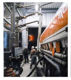
EMCO bottom loading achieves easy filling of tank trucks. Simultaneous loading of 5 different products is possible. No matter, where you want: Premium in the front, Unleaded in the middle and Diesel in the rear, EMCO bottom loading gives you total flexibility.
