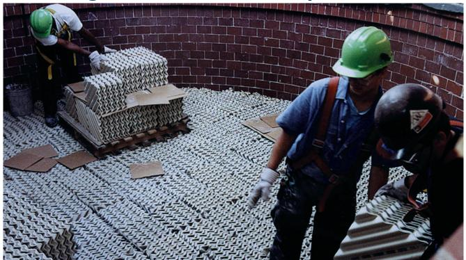
Koch Knight LLC can put it all together for you from process design and mechanical layout to field construction and installation.
