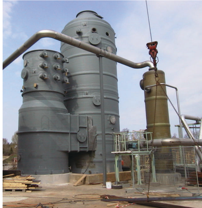
GRP Flue Gas Condensing Scrubber
