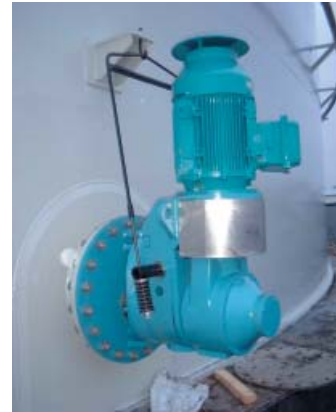
Plenty swivel angle gear drive mixer in a Russian oil refinery
