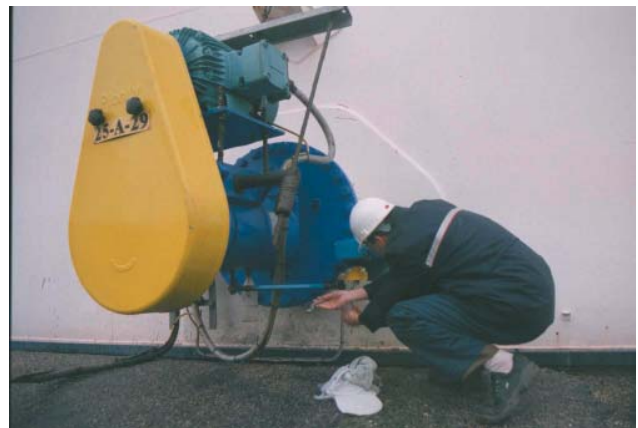
Final installation of a Plenty belt drive mixer
