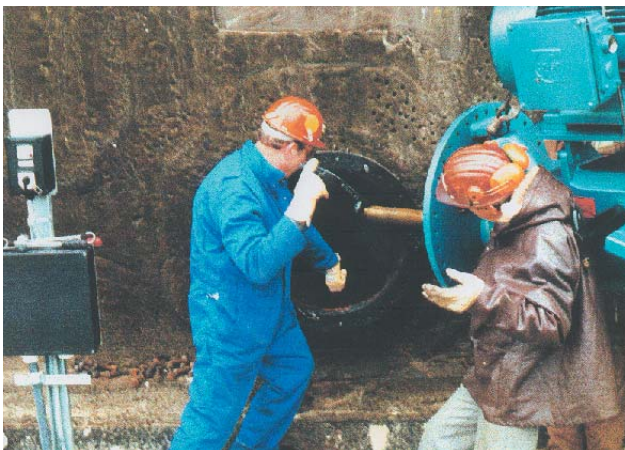
Installing a Plenty belt drive mixer in Europe
