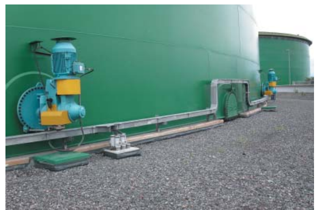
Plenty swivel angle belt drive mixer complete with automatic actuator
