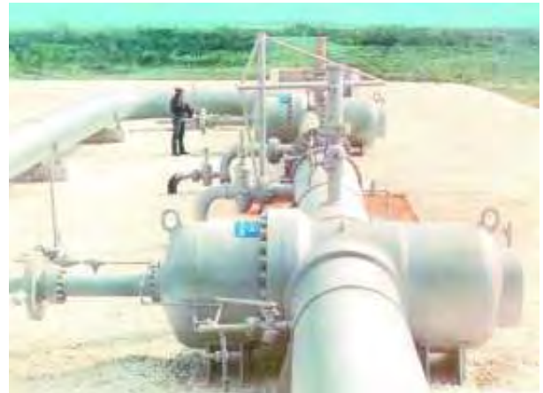
WKM Model G Series Pow-R-Seal Gate Valve in a block valve application on a pipeline loop - possibly a pigging loop. Note smaller WKM Model D Pow-R-Seals possibly used as "kicker valves"
