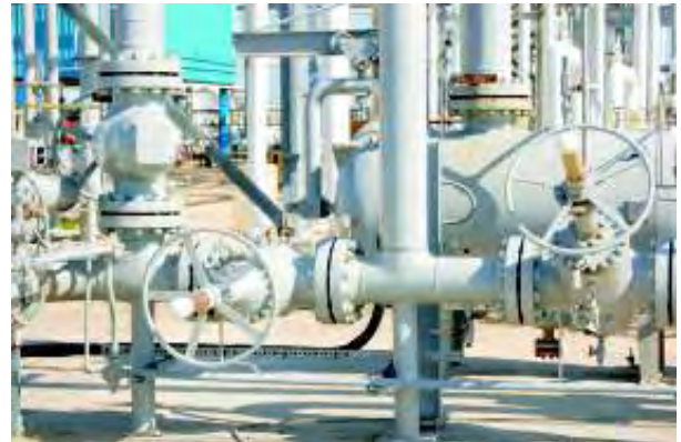
WKM Model E Pow-R-Seal Gate Valves on the inlet to a gas sweetening plant
