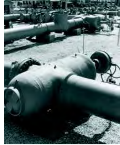
WKM Model D Pow-R-Seal Gate Valve acting as a block valve in a pipeline expansion
