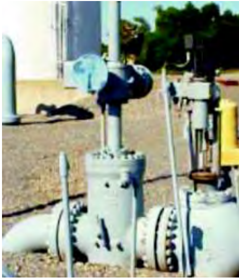
WKM Model E1 Pow-R-Seal Gate Valve used for isolation of a control valve in a liquids pipeline
