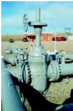
18 inch (450 mm) 600 WKM Model E Pow-R-Seal Gate Valve in a block valve application
