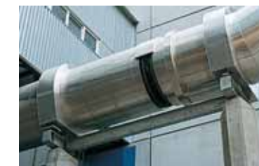
AC1 joint with weather cap
