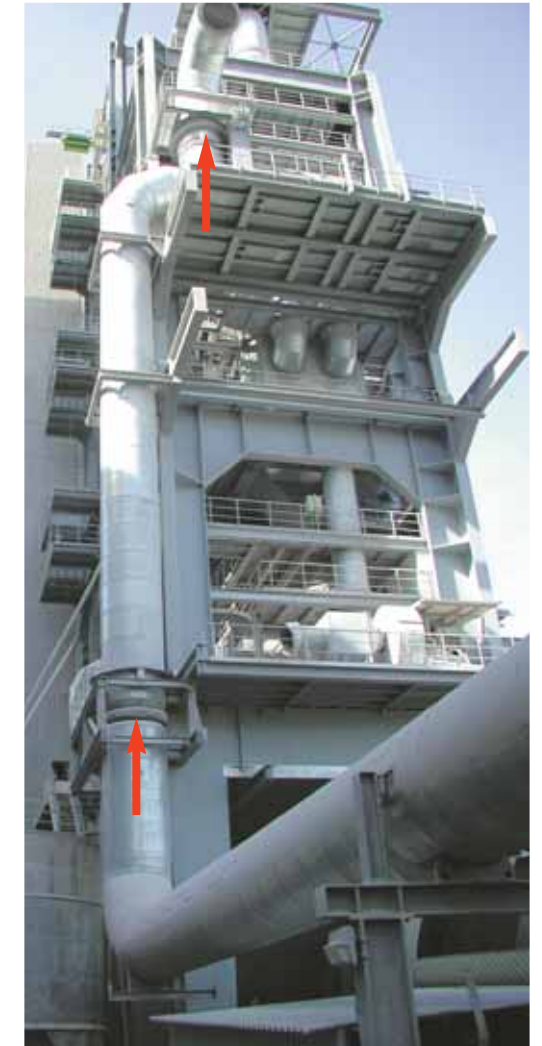
KOREMA® joints in a typical ducting run for a cement plant
