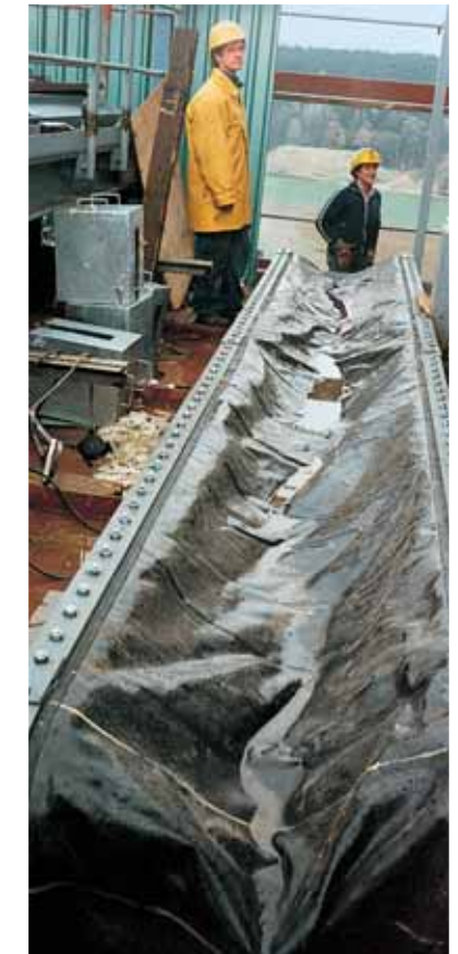
On site installation
