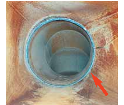
SIMIFLON® expansion joint in a garbage incinerator duct
