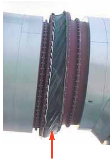
Cement plant – expansion joint with lateral preset
