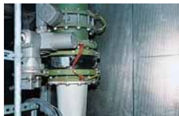
Expansion joint with static protection
