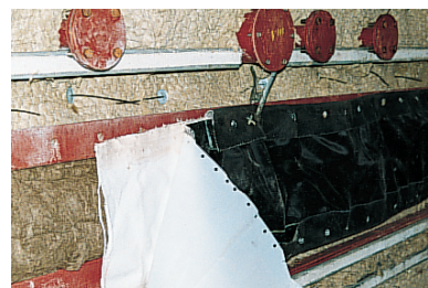
6. Assembly of the multilayer expansion joint.
