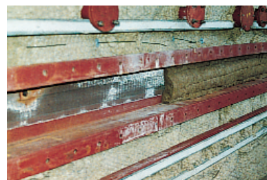
4. Mineral wool is installed.
