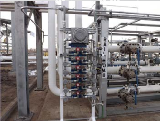
Additive Injector Install— Hammond, Indiana
