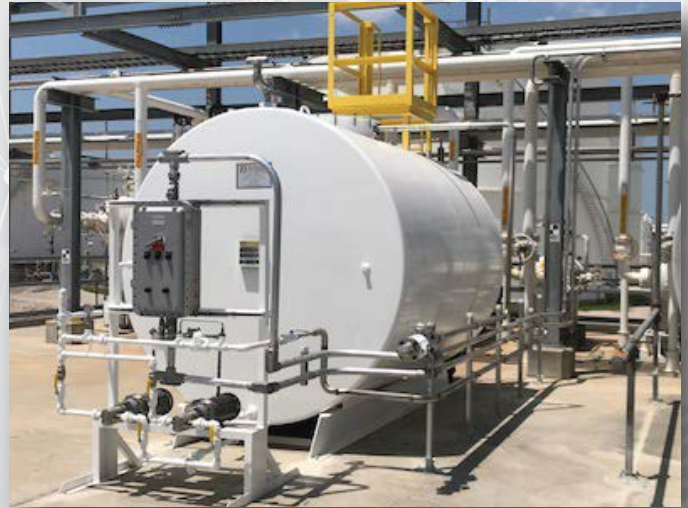
4K Tank w/ Dual Pump Skid Install - Corpus Christi, TX
