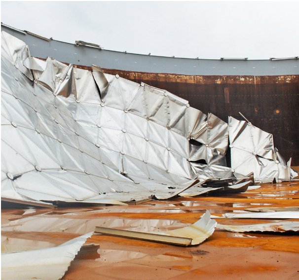
Figure 2. Full consideration of local regulations with the dome's custom configuration regarding the geographic location can ensure the aluminium dome roof will withstand environmental conditions; not doing so can be catastrophic.
