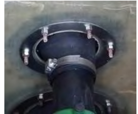
4-Bolt Nupi Fitting Example
