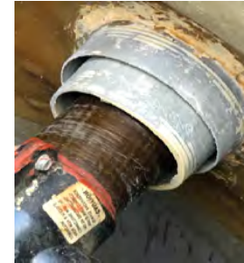
Example of Western Fiberglass Double-Wall Cuff Fitting
