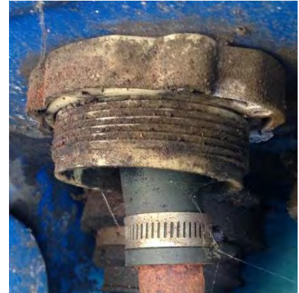
Example of TCI Direct Bury Fitting
