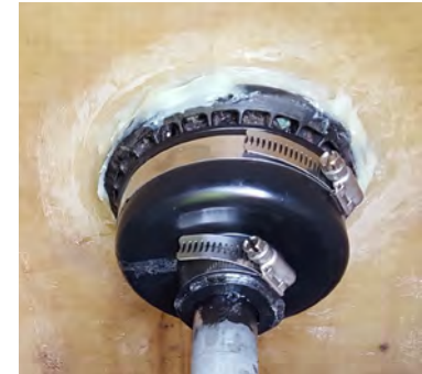
Example of Blueline Small KFD Repaired
