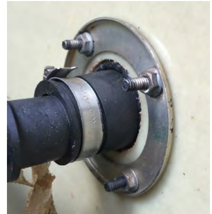
4-Bolt OPW Fitting Example
