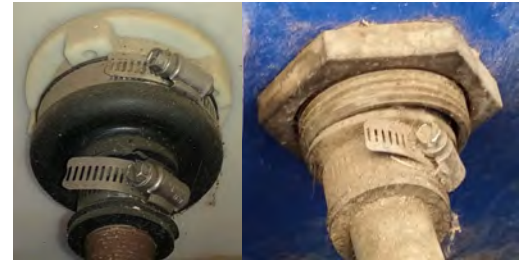
Examples of TCI Conduit Fittings
