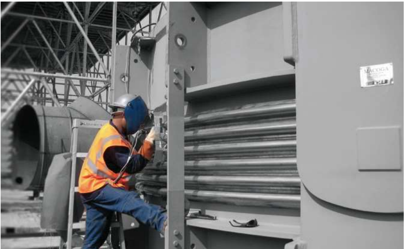
Assembly of a 7200 mm diameter MUX Expansion Joints in a Power Plant in Turkey
