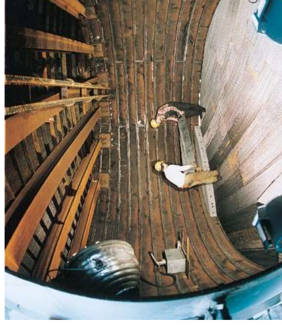
Installation of Montz-Pak Type B1-300 into a column DN 5600 from which the existing valve trays have previously been removed. All supporting rings have been removed by torch-cutting.
