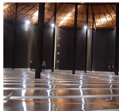
Heavy duty IFR fully assembled and installed.
