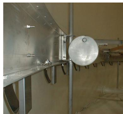
310mm deep extruded channel rim is strong enough for the Matrix Applied Technologies IFR shoe seal to be connected to it without additional bracing.
