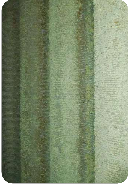
Before cleaning the uppermost bank economiser
