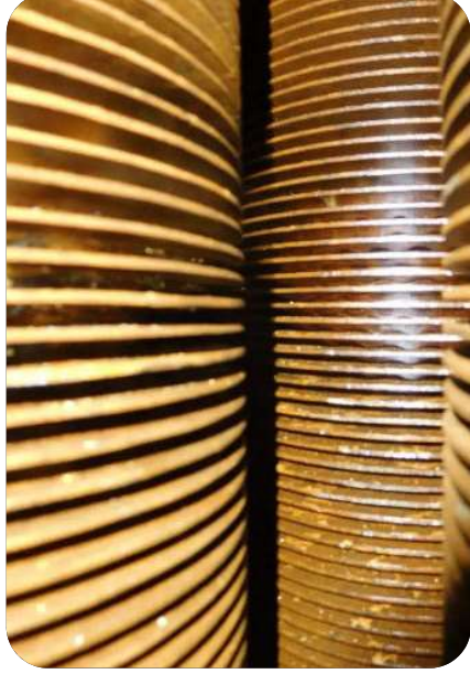
After cleaning the uppermost bank economiser
